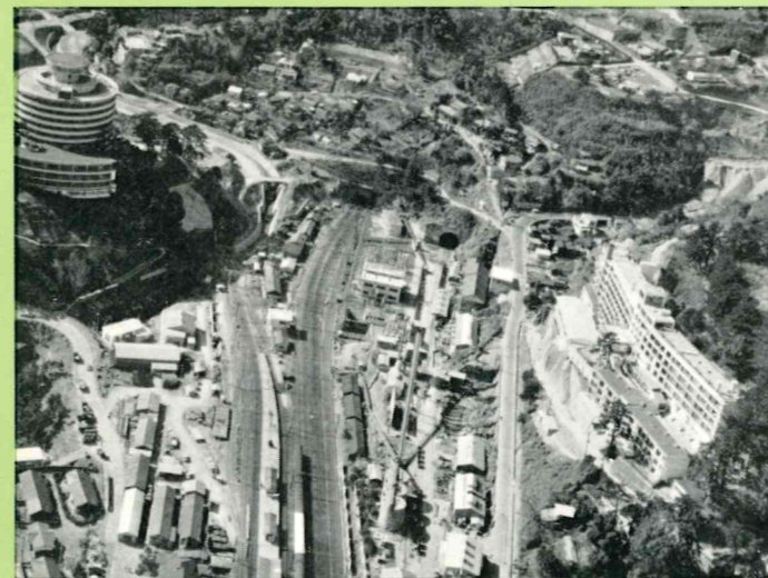
New Tanna Tunnel under construction
