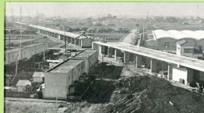
Rails just ready to be laid (near Odawara)
