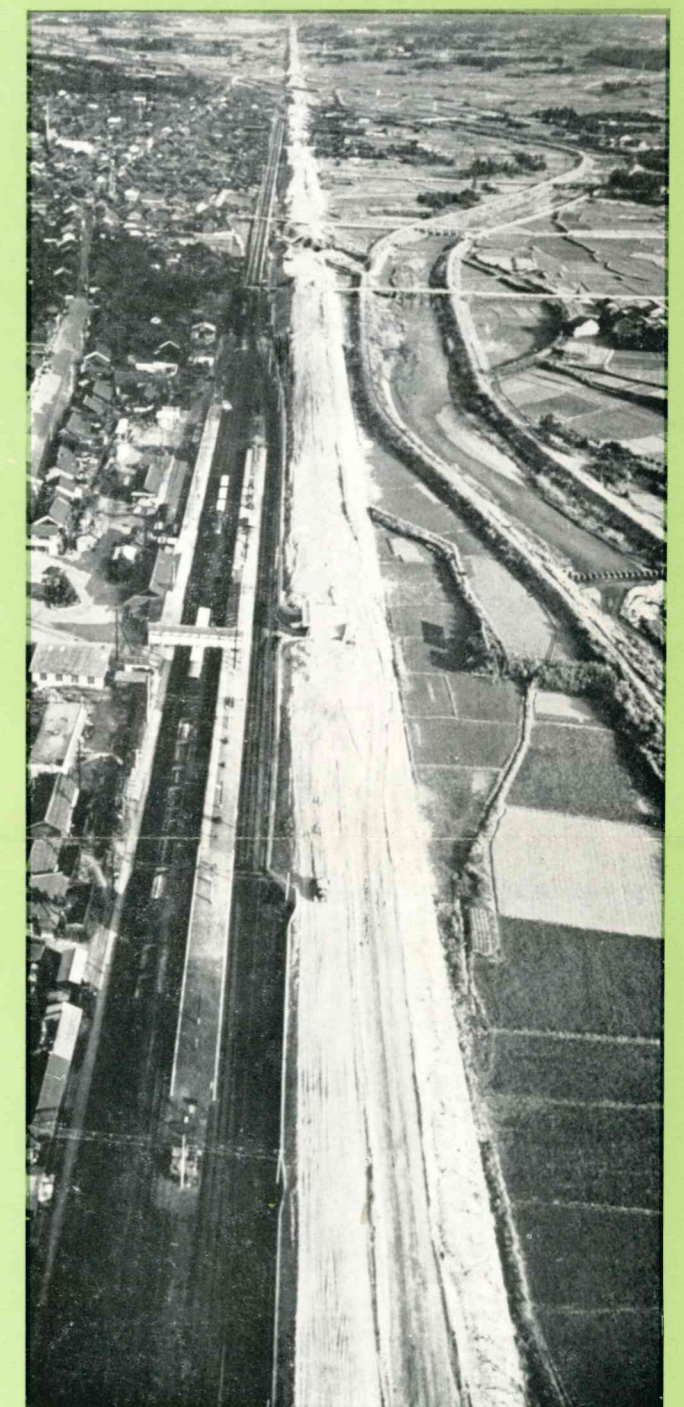
Earthwork at Futagawa (near Toyohashi)
