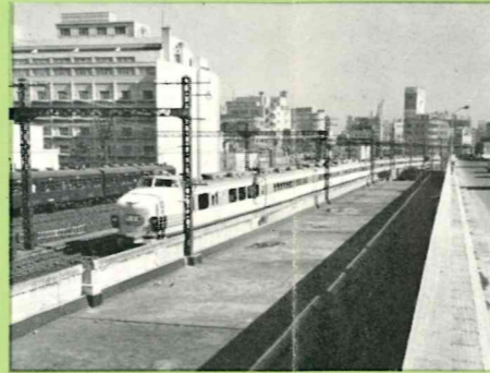
Elevated track bed outside of Tokyo Station
